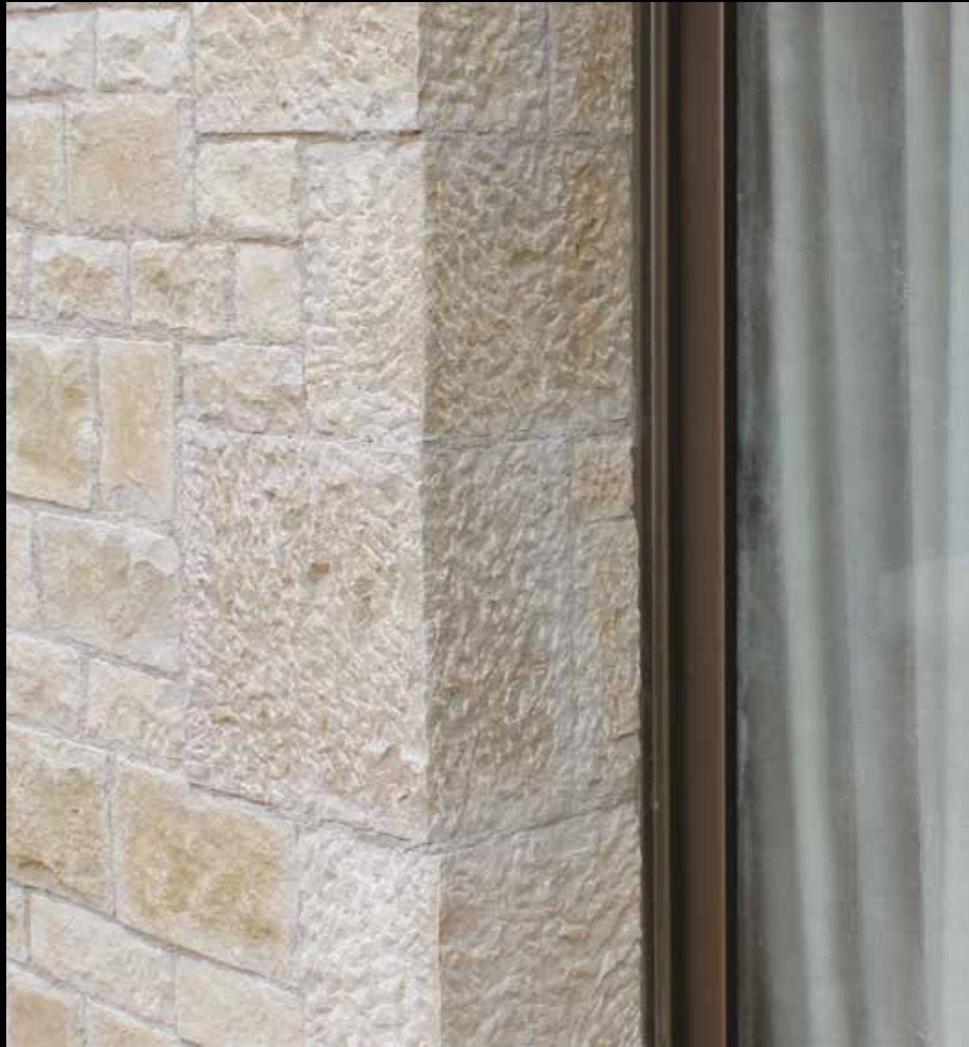
Posedano Corner detail
