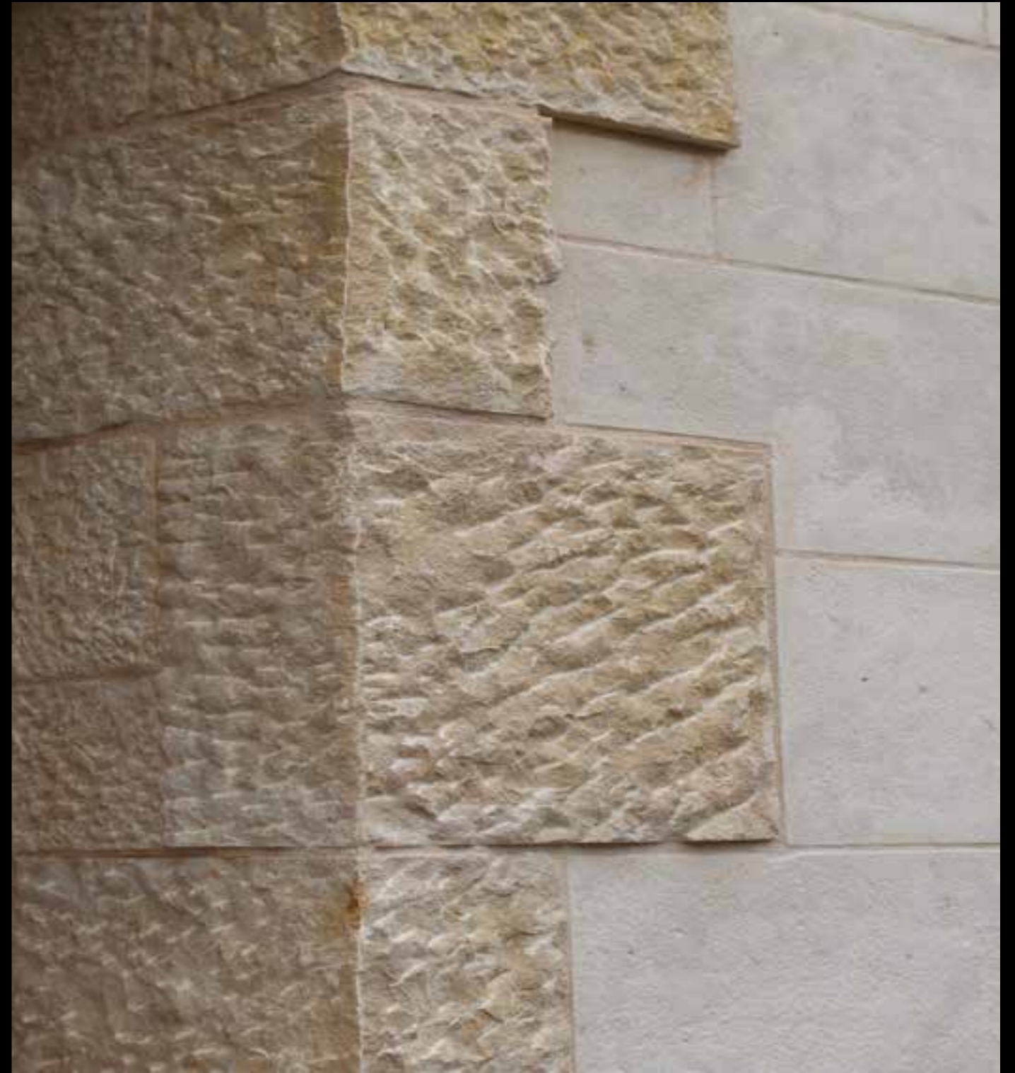
Posedano Corner detail
